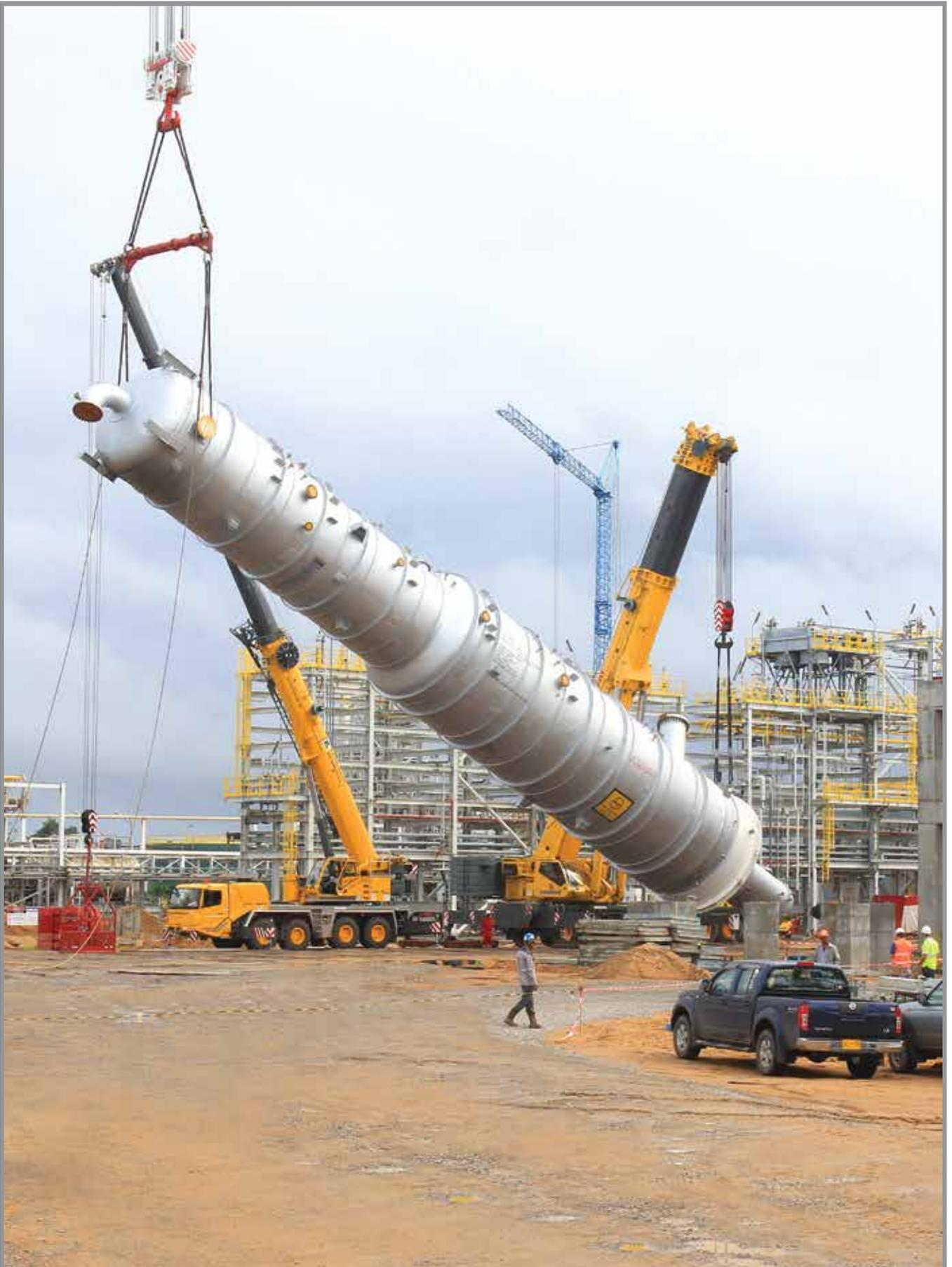
Work in progress at the Refinery Expansion Project. The vacuum tower is placed on its foundation.
