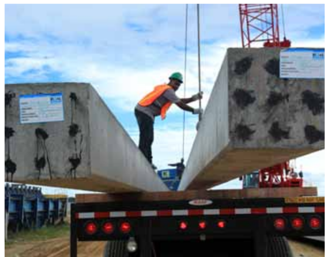
Transport of material and equipment.
