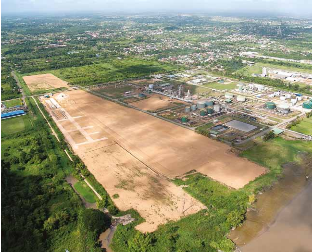
The site where the new refinery is being constructed.
