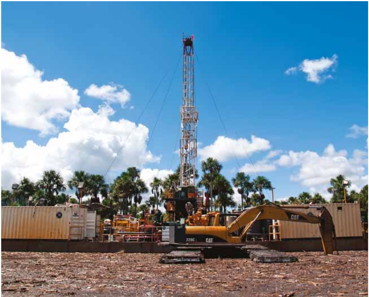
A rig in the swamp area of the Coronie block.
