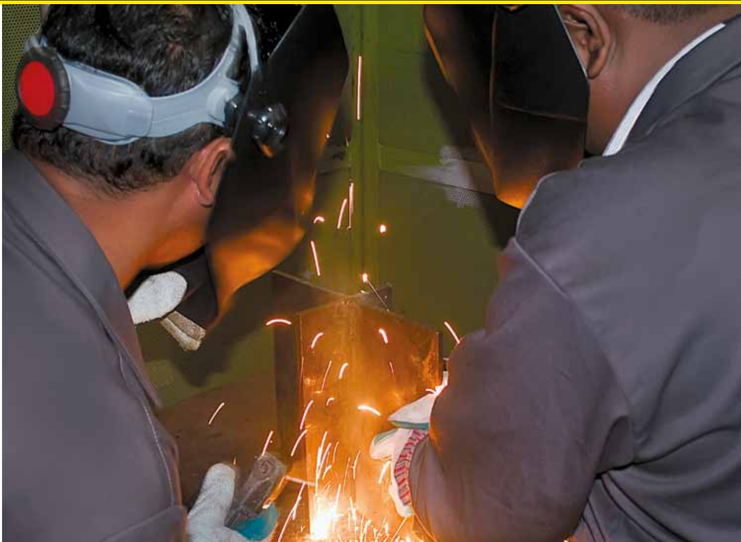
Certified welders will be employed for the construction of the new refinery
