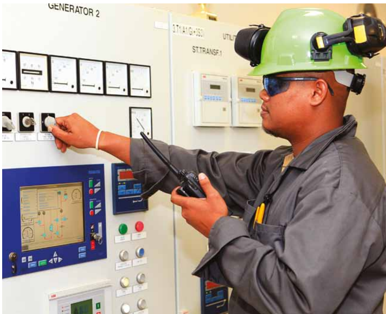
The control room of Staatsolie Power Company Suriname
