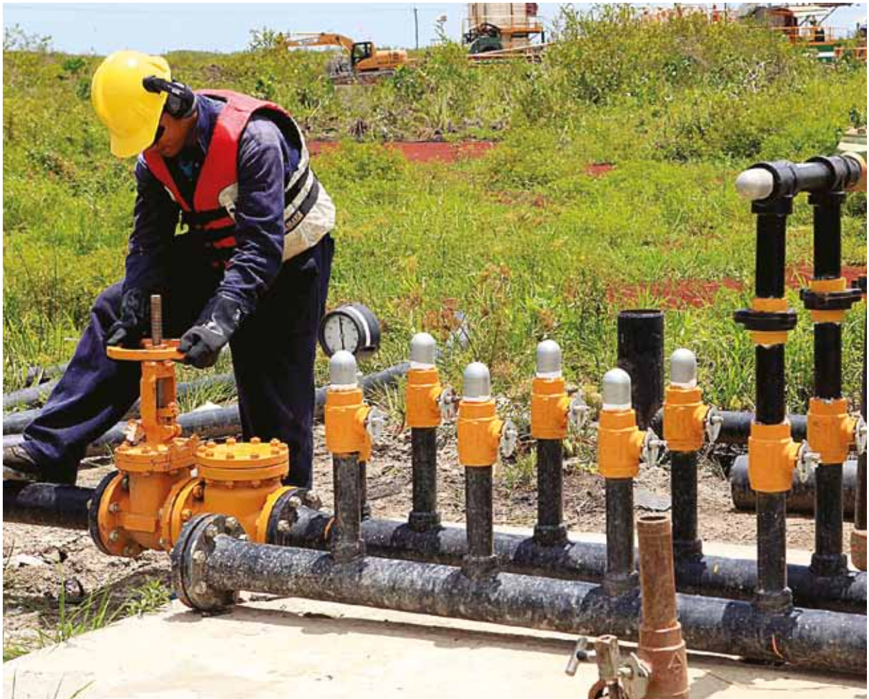
Opening a valve on a main line in the Tambaredjo oil field as part of the commissioning of a manifold, where new sources are connected.
